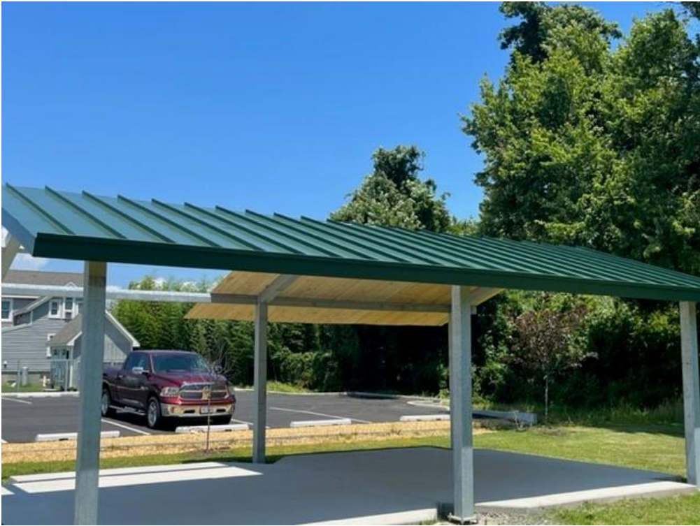
BKP Pavilion Roof
