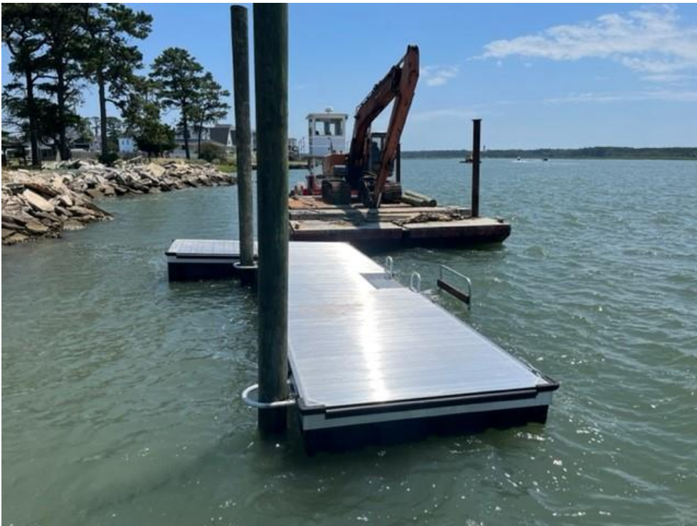
Kayak Launching Facility at Memorial Park
