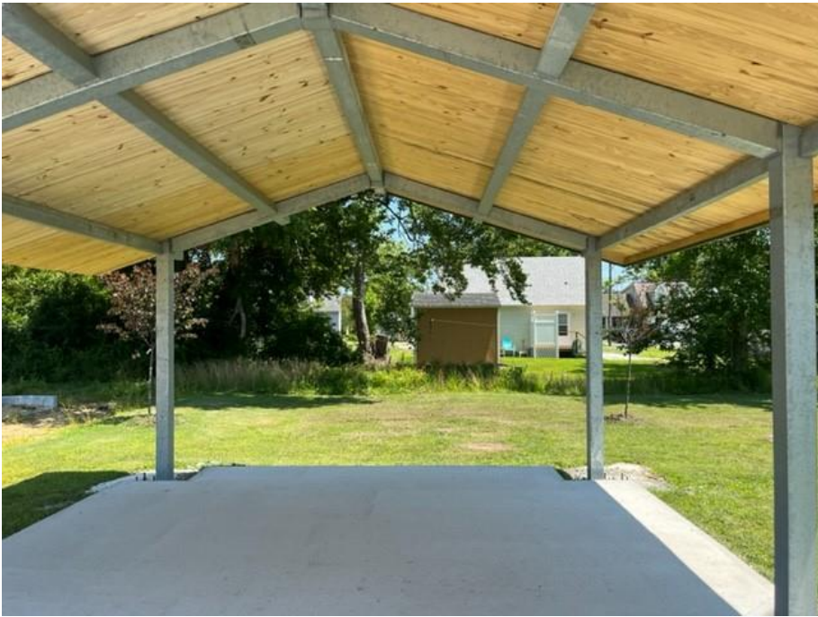
BKP Pavilion Roof
