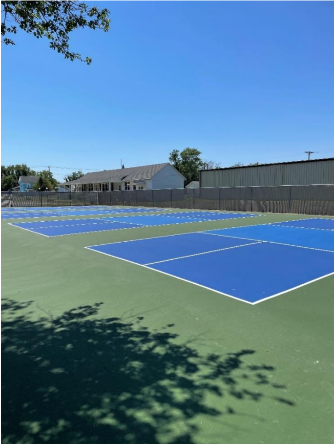
New Pickleball Courts and Fence
